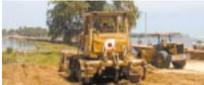
Road rehabilitation work
